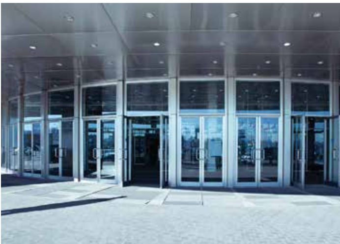
Front Entrance facing south
