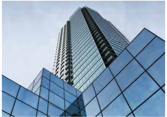
Exterior Rear facing northwest
